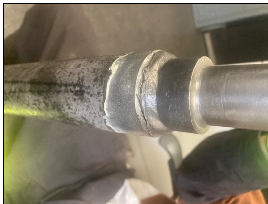
Figure 3: Cracked weld at pin/tube joint weld
